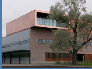
Aurora 2, Joensuu university building 8,100 m 2 2006 202 kWh/(m 2 a) 1) The building is U-shaped. There are glazed courtyards for the distribution of daylight to the surrounding office spaces in both wings.
