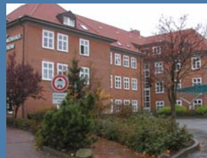
District, Hagenow Hospital 16,000 m 2 1994 210 1) kWh/m 2 155 2) kWh/m 2
